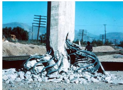
Failed bridge column as a result of the 1971 earthquake San Fernando Valley, California
