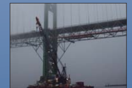
Serenity image belies rapid progress. Whether working in rain or shine, crews forged ahead to complete construction on both caissons by summer 2004. Derrick barges provided work platforms for crews, equipment and supplies. Fall 2003
