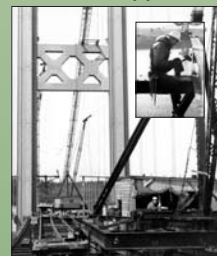
Bracing against the elements. The 33-foot deep Warren truss system was assembled at the bridge site from shop-fabricated components. Four rolling derricks (2 per tower) moved each way from the towers. Two nesting cranes and traveler operators worked from the lower piers to the center of the main span, while two other crews worked from
