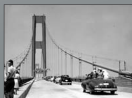
Opening day, July 1, 1940. At the opening ceremonies, several bands played a march composed by the Gig Harbor postmaster. The bridge cost $6.4 million; tolls started at 55 cents and were cut to 50 cents two months later when the bonds were refinanced.
