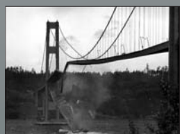
Thursday, November 7, 1940. For bridge engineers, it's a day that forever lives in infamy. Just four months after the span opened to traffic, it tore apart in a 40-mile-per-hour windstorm. At about 10:30 a.m., a center span floor panel dropped into the water 195 feet below. The roadway broke up and chunks of concrete and steel pelted the Narrows. Galloping Gertie's demise may represent the most dramatic failure in the history of bridge engineering. But it's a failure that has contributed significantly to the design and construction of the second, remarkably stable suspension bridge of today.
