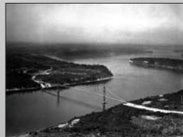
The Narrows and Lady Gertie. Construction of the first bridge began November 23, 1938. Workers completed the bridge in only 15 months as compared to the 29 months it took to finish the 1950 (existing) bridge.
