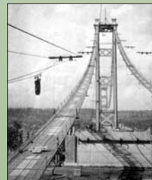
Cables & Spinning. Once the towers and cable saddles had been built, the main suspension cables. Spaced 60 feet apart, each cable contained 19 strands of 458 No. 6 gauge wires.
