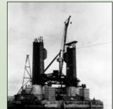
New bridge built on 1940 piers. Engineers faced two major challenges in building the second bridge. First, they had to understand the failure of the 1940 bridge, and then design a new one to withstand the same conditions. Next, they had to determine if remnants of the old bridge — the lower foundations — could be used. The two foundations were undamaged and were used to support the second bridge with only minor modifications.
