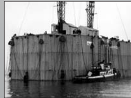
1940 caisson lags in place. The bridge foundations for the first bridge were used to support the towers of the present-day bridge built in 1950.
