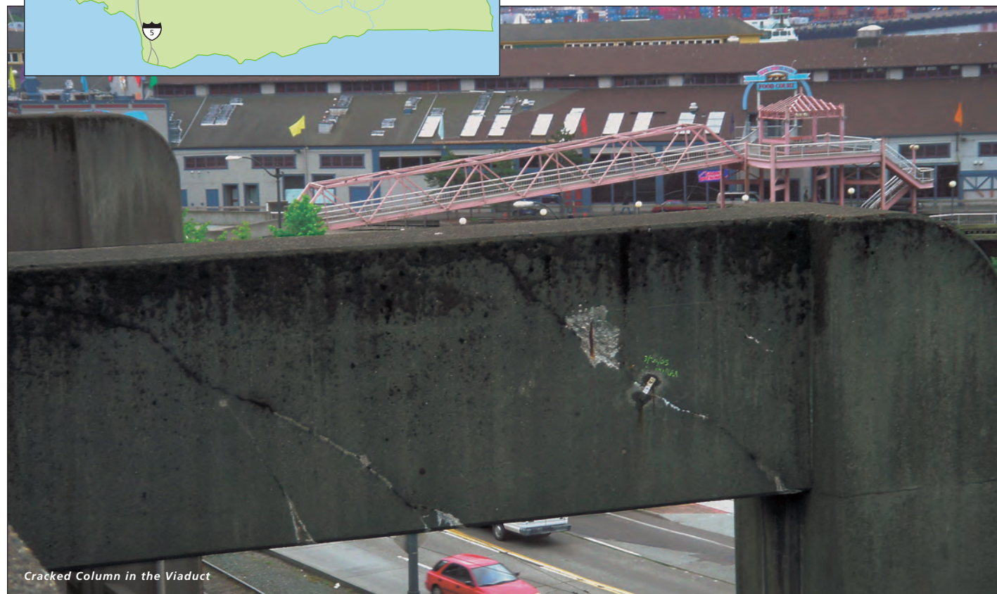
Damaged Rebar in the Viaduct
