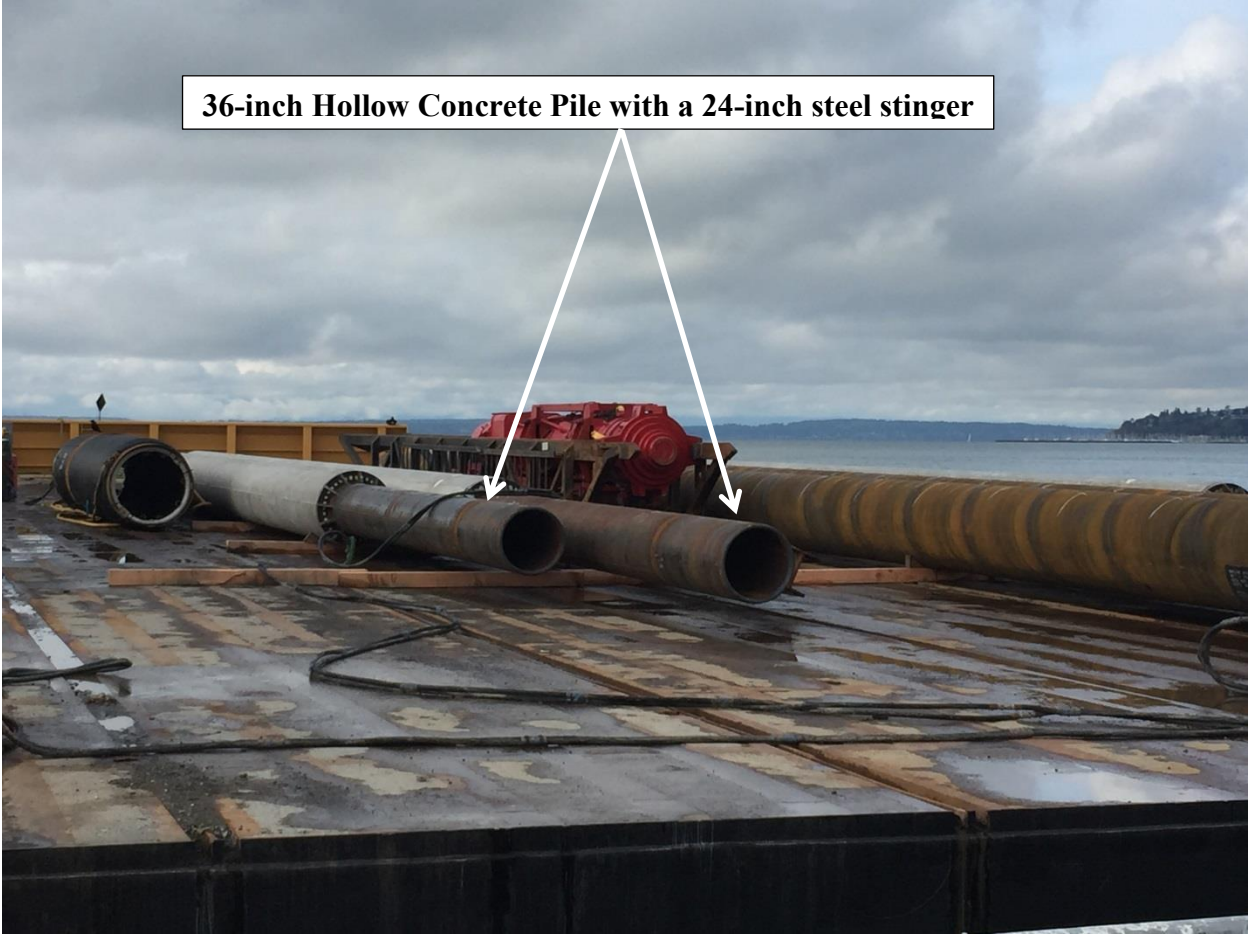
Figure 5: 36-inch Hollow Concrete Pile with a 24-inch steel stinger
