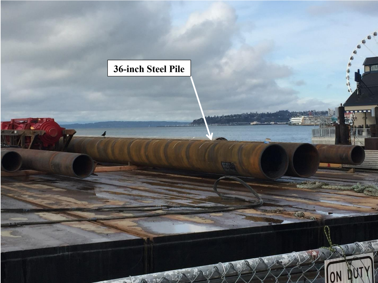
Figure 4: 36-inch Steel Pile
