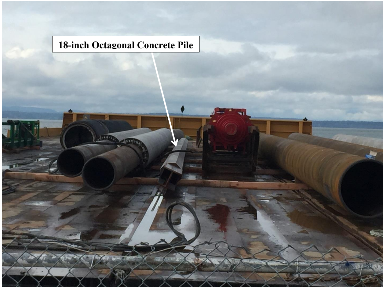
Figure 6: 18-inch Solid Octagonal Concrete Pile with a 12-inch steel stinger
